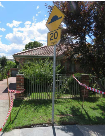
Photo 1: The energised street sign
