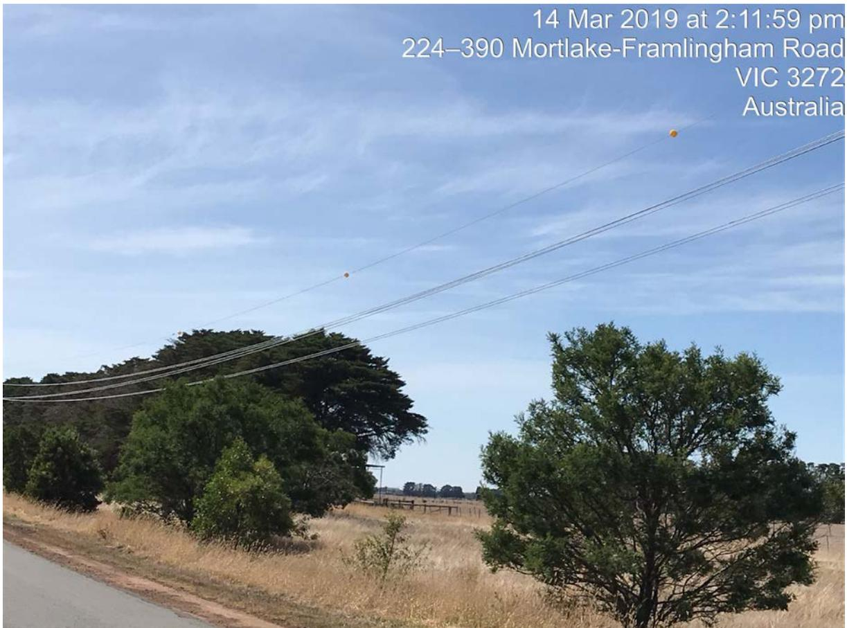
Photo 2: Three marking balls on one span
