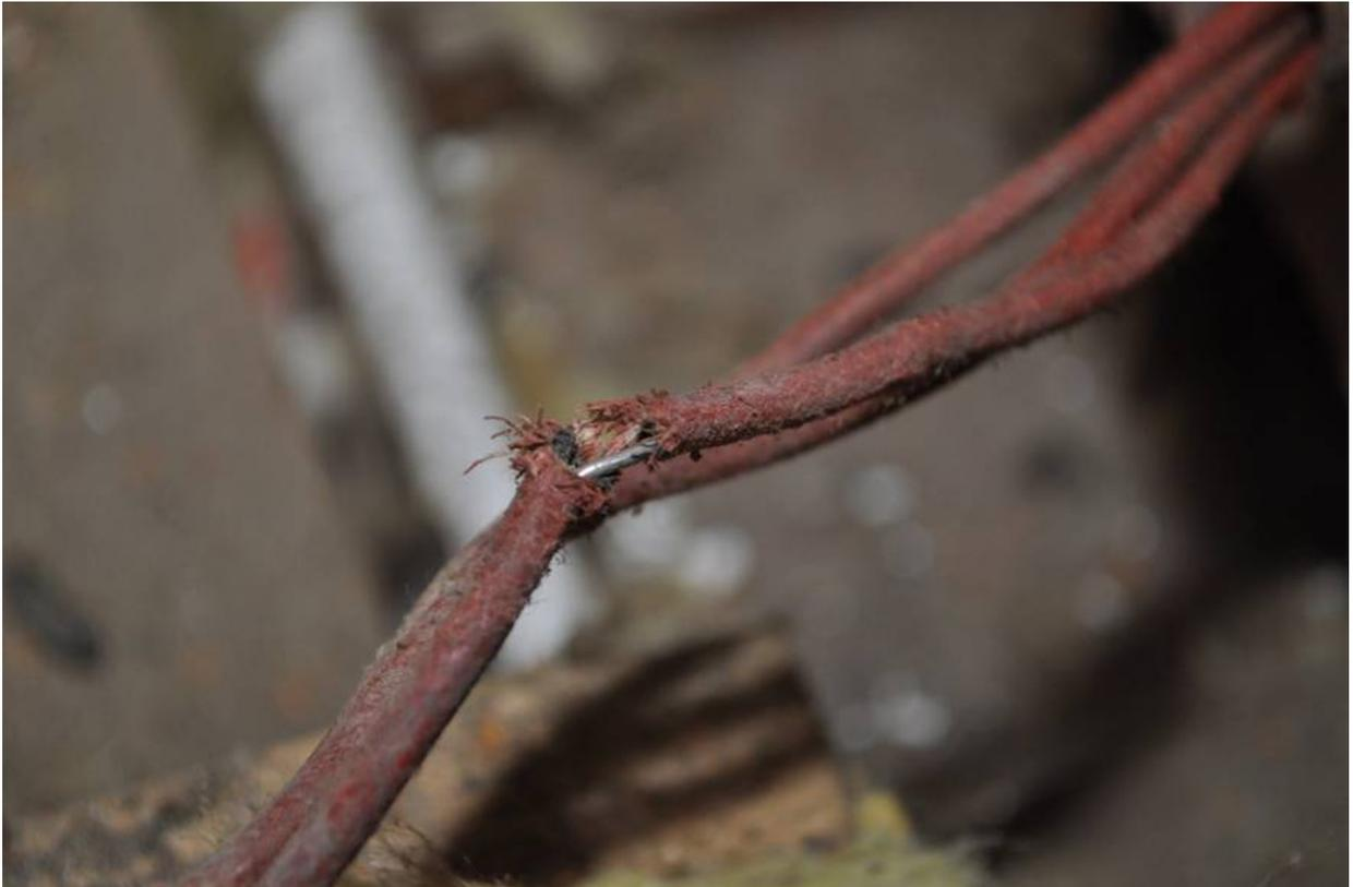
Picture: Old, degraded household wiring like this can cause fires and electrocution.
