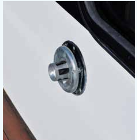
Figure 15 and 16: Flue terminal for IHWS (left) and space heater (right)
