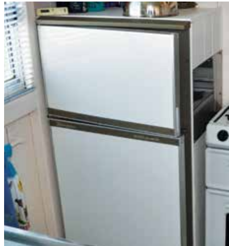
Figure 13: LPG refrigerator installed in a recess
