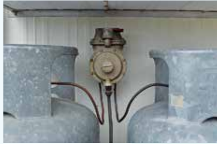
Figure 6: This is an example of a non-compliant installation. Liquid gas can not drain back into the cylinder due to the position of the gas pipes.
